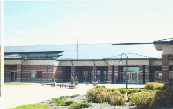
The recently built Perrysburg High School.
